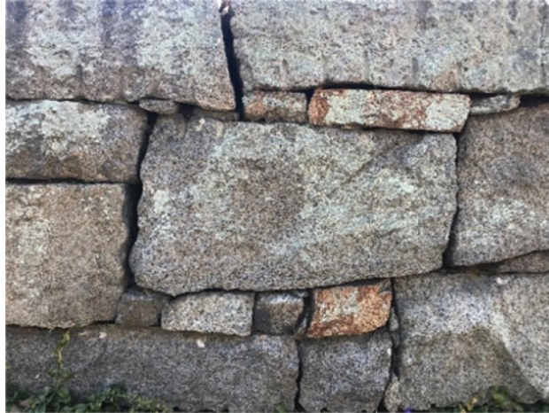
FIGURE 3 | Cut granite wall.
