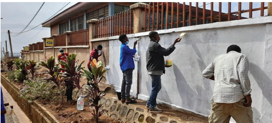
FIGURE 10 | Applying white Pantex (paint) on the wall.
