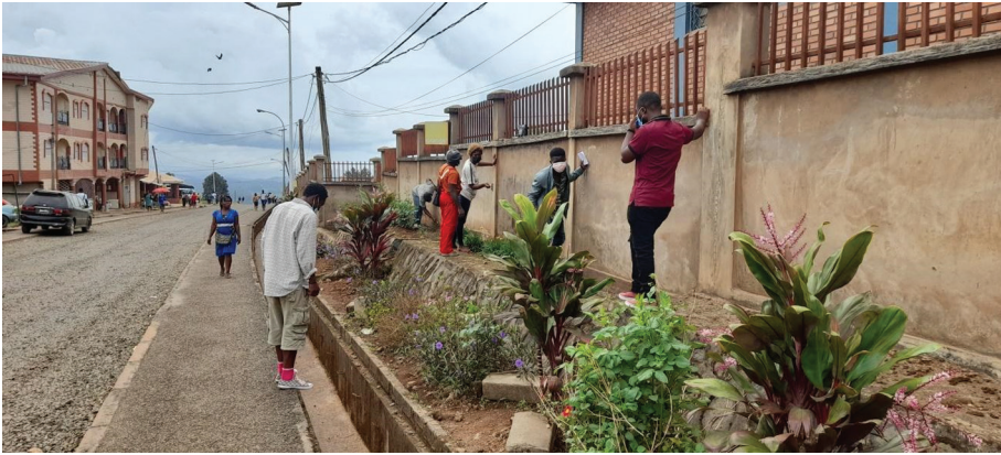
FIGURE 8 | Students removing dirt from the wall surface to be painted.
